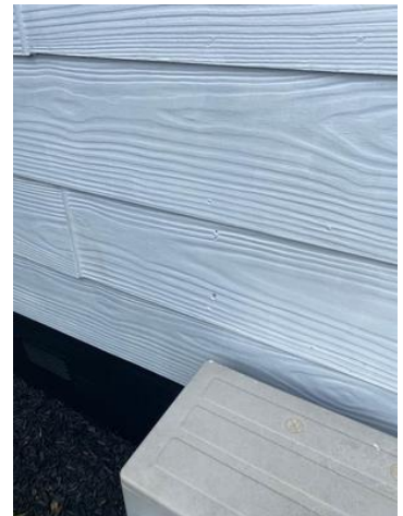
Small holes to cladding.
