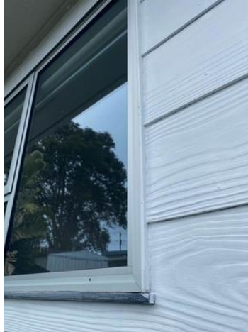
Recommend ensuring good seal to side of windows.
