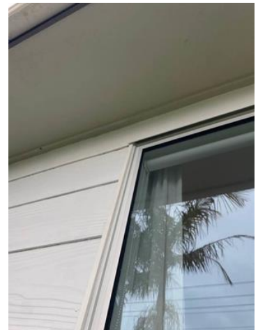
Side of window well sealed.
