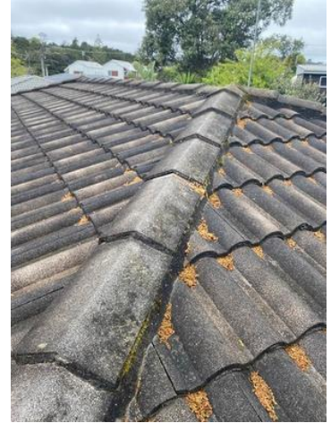
Cracked and missing pointing.
