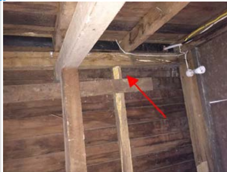
Bearer over span. Has props which go to ground.
