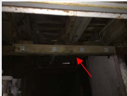
Flitch plate to bearer below joists
