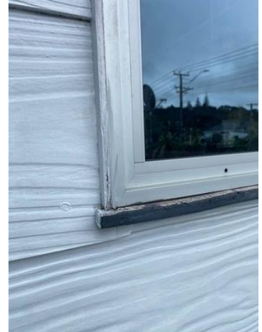
Some deterioration to sill and scribes.
