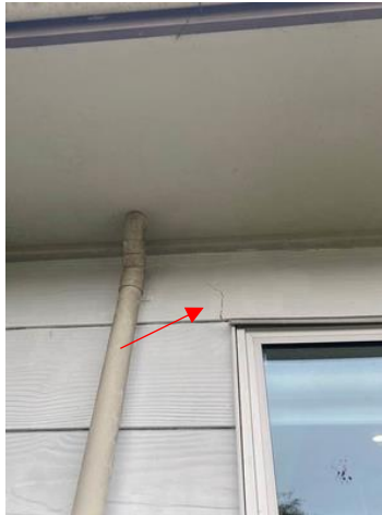
Crack to cladding.
