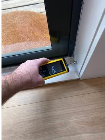
Significant unevenness to the floor to this area.
