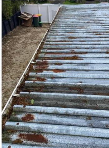
Corrosion to shed roof.
