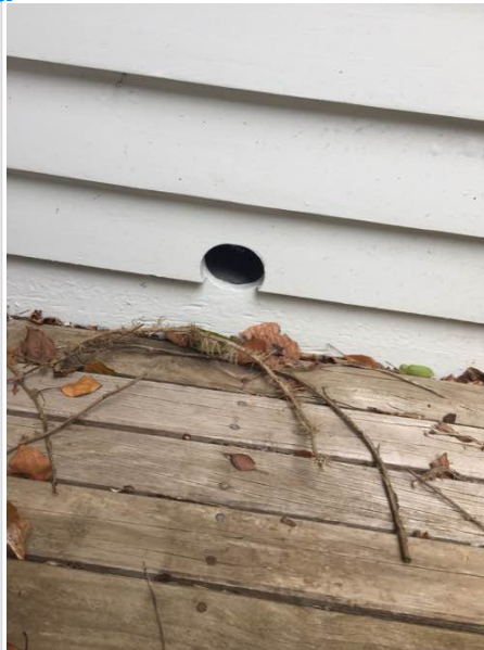
Hole to cladding should she sealed
