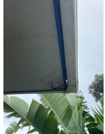
Moisture damage to soffit.
