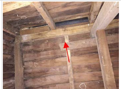
Bearer is over span.
