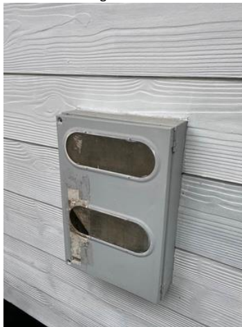
No head flashing. Appears well sealed.
