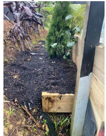
No drainage to rear of wall.
