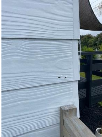
Holes to cladding. Require sealing.
