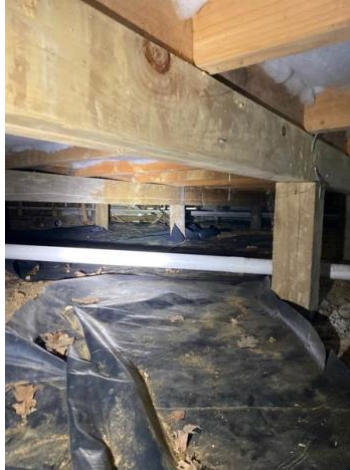
Inadequate ground moisture barrier.
