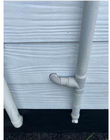
Penetration requires sealing.
