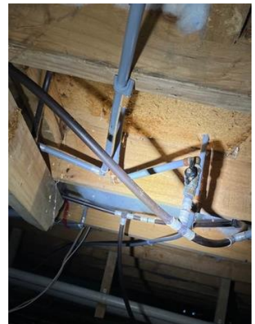
No visible leaks. Some moisture staining to particle board.
