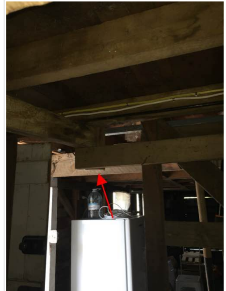
4x2 canitlevered stringer holding up a bearer over the extension
