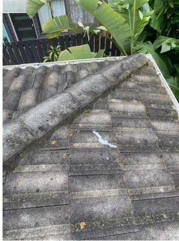
Silicone repairs.
