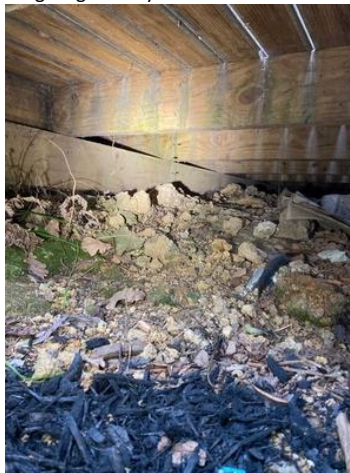
Bearer in contact with ground. Incorrect treatment.
