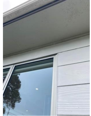
Minimal cover to head flashing.
