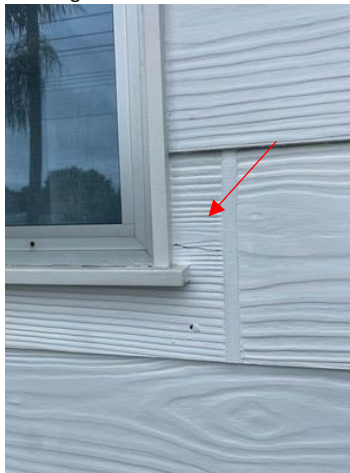
Crack to cladding.
