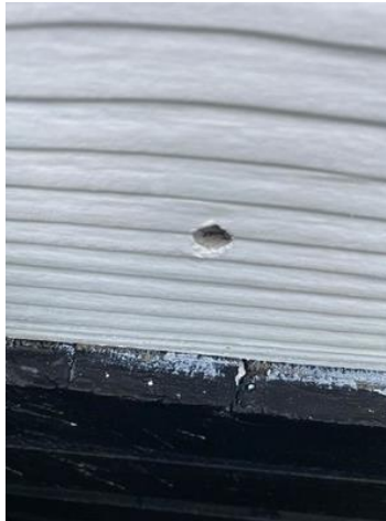
Cladding is fibre cement.
