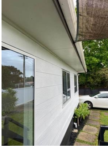
Height of windows in relation to soffit overhang good.
