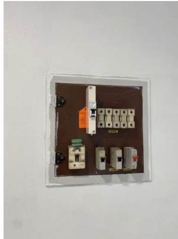
Older style switch board, no RCD protection.
