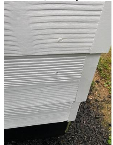
Recommend sealing hole.
