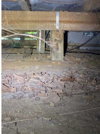
Piles and bearers appear in good condition.
