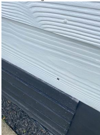
Recommend sealing hole.
