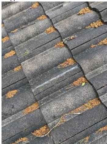
Silicone repairs to tiles.
