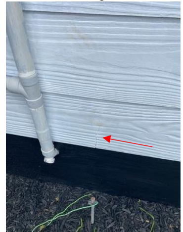
Crack to cladding.
