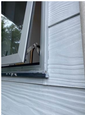
Recommend ensuring good seal to side of windows.
