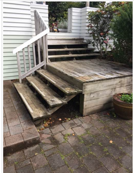
Timber to landing appears to be of correct treatment.
