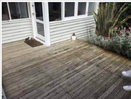
Main deck is in average condition
