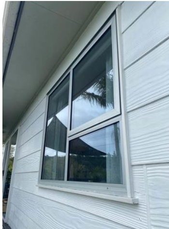
Retrofitted double glazing.
