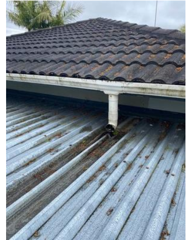
Recommend installing spreader.
