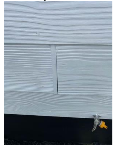
Gaps to jointer. Recommend sealing.
