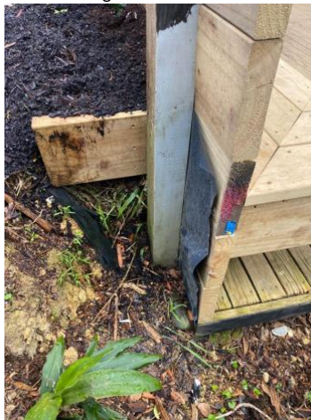
Incorrect timber treatment to retaining wall.
