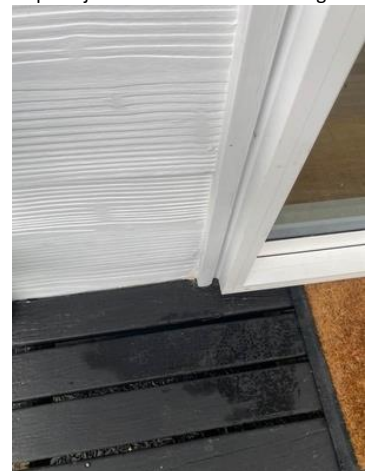
Damage to base of cladding.
