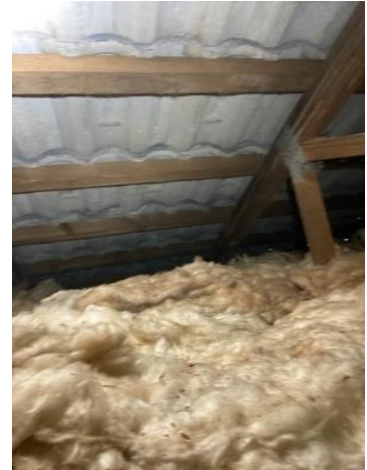
Insulation has a good, snug fit.
