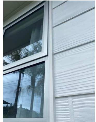
Side of window well sealed.
