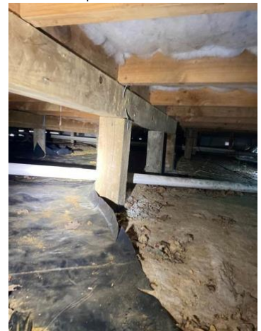
Pile to bearer connection.
