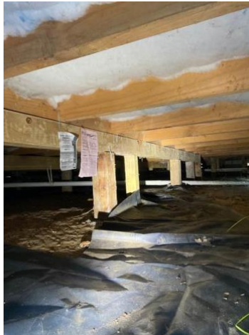
Insulation of the correct 'R' rating.
