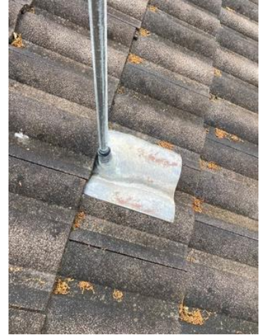
Recommend ensuring good seal to penetrations.
