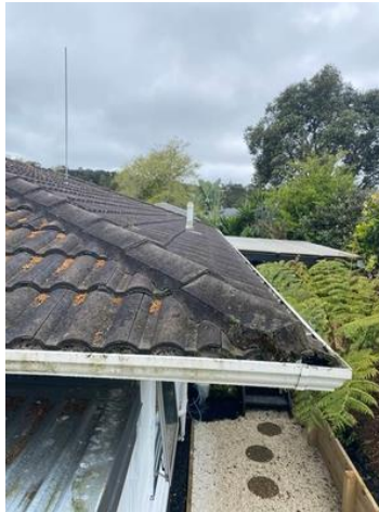
Cracked and missing pointing.
