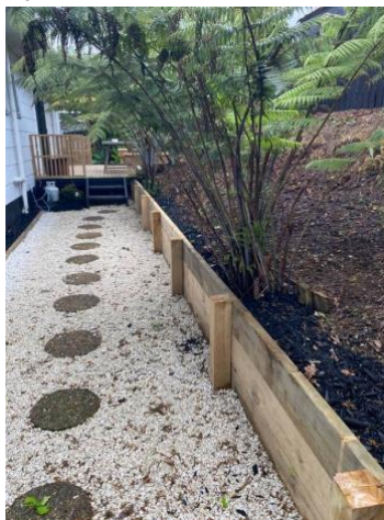
Incorrect treatment. Wall on slight lean.
